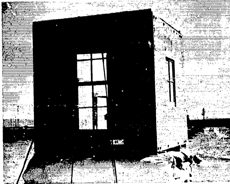
Fig. A.4. Room at 7000-ft Station Before Shot 3.
